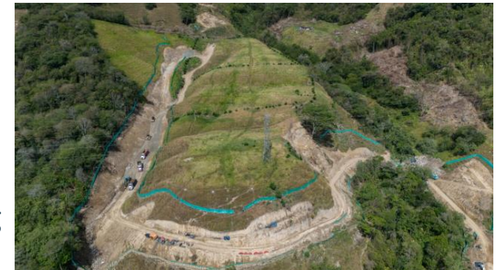
Access road construction progress at Marmato Lower Mine
