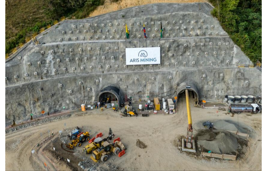
Process plant foundation earthworks 12% ahead of schedule as of the end of February 2025
