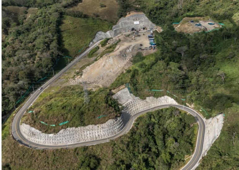
Access roads to the Lower Marmato process facility and accommodation camp now 100% complete
