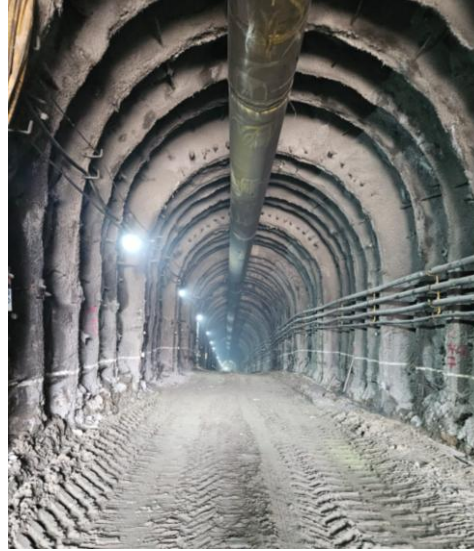
Decline development underway with 200 metres completed to the end of February 2025
