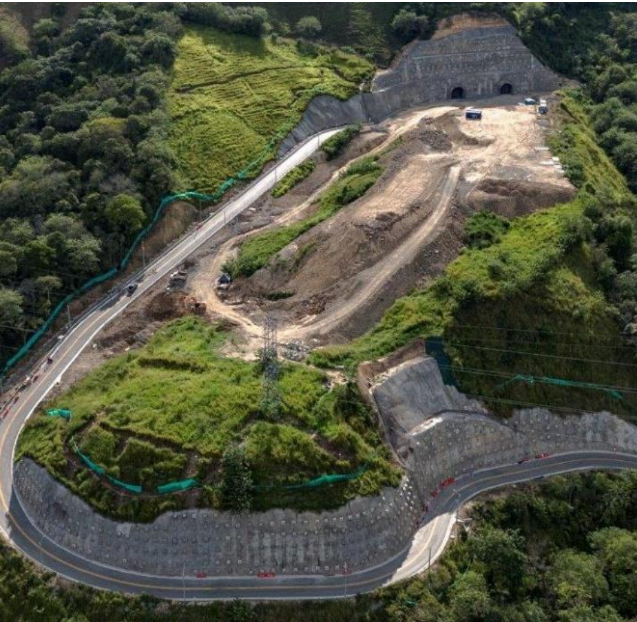
Road Access and Plant Platform
