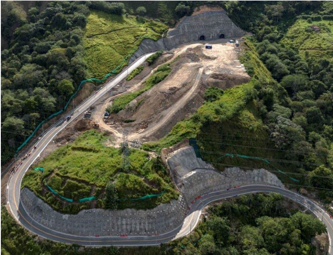
Road Access and Plant Platform
