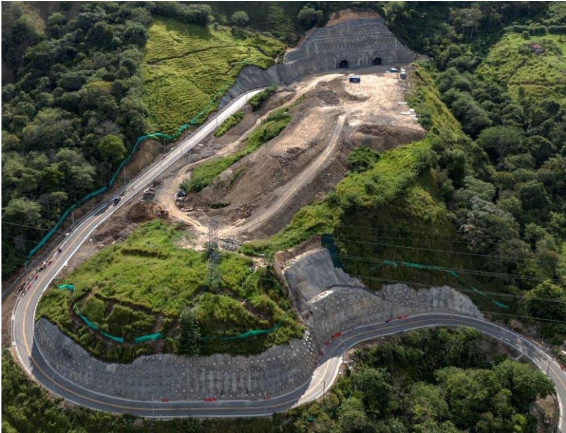
Road Access and Plant Platform
