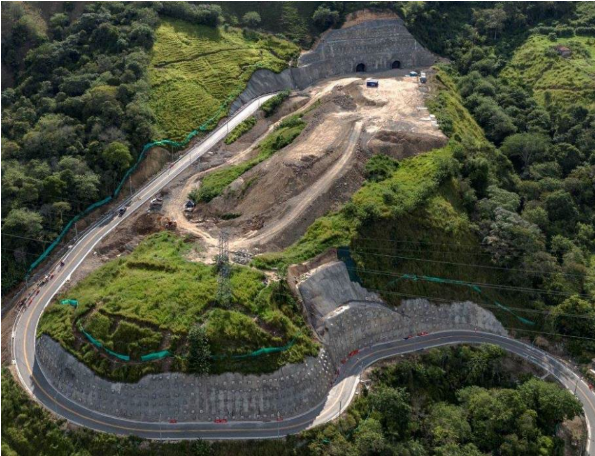
Road Access and Plant Platform
