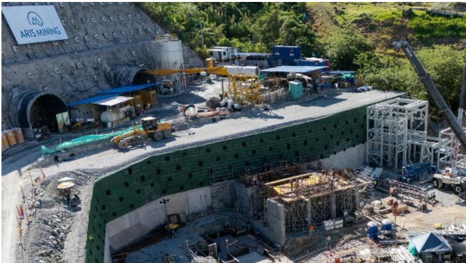
Crusher area moving into mechanical installation
