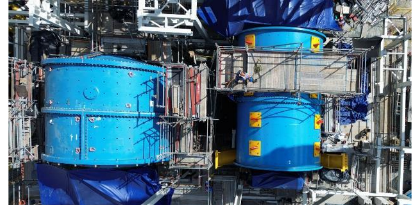
July 27, 2026: Installation of SAG and ball mills
